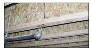
**Large Drop**. Deflectors may be installed 1 to 6 inches below the bottom of the joist as long as the distance between the sprinkler and ceiling does not exceed 22 inches. Firestopping is not required because large drop sprinklers are limited to a protection area of 100 sq. ft. and a maximum spacing of 10 feet.
