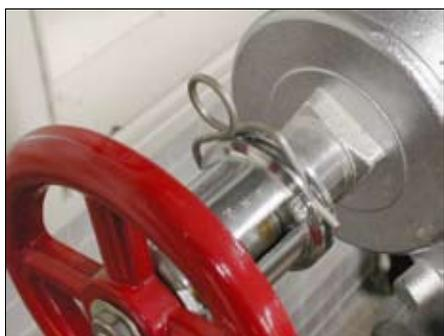
There are two methods of setting outlet pressures: **field set** and **factory set**. Field-set devices are designed and manufactured so their pressure settings can be adjusted after the device is installed on the standpipe riser. This gives the installer the greatest amount of flexibility to install the devices at any location and adjust them later.
