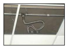
The number of bends may be limited by the manufacturer, and minimum bend radius must be 3 inches (7.62 cm). Once installed, these sprinkler drops should be pneumatically and/or hydrostatically tested in accordance with regular sprinkler system test procedures. The maximum rated pressure for these items is 175 psi (1205 kPa).
