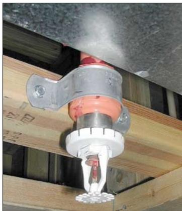
A representative sample for testing is at least four sprinklers, or 1 percent of the number of sprinklers per individual sprinkler sample, whichever is greater. Where one sprinkler within a representative sample fails to meet the test requirement, NFPA 25, *Standard for the Inspection, Testing, and Maintenance of Water-Based Fire Protection Systems*, requires that all sprinklers represented by that sample shall be replaced.
