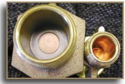
The photograph illustrates the orifices of two sprinklers: an Early Suppression, Fast Response (ESFR) on the left, and a standard spray sprinkler on the right. The ESFR has a K factor of 25.2 and the standard sprinkler has a K of 5.6.
