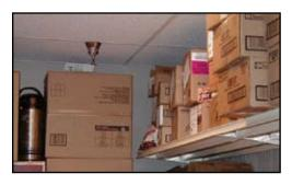
NFPA 13 allows less than 18 inches clearance from ceiling sprinklers when large-scale fire tests for the particular hazard show less clearance is acceptable.
