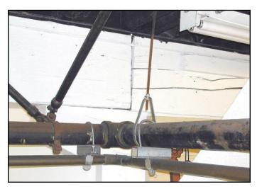
Because they often are exposed and a convenient size, sprinkler pipes get used for storage racks, clothes hangers, electrical conduit supports, telecommunication or power cable hangers, or tool brackets. Not only do these loads put additional stress on the hangers, but they may create obstructions to sprinkler discharge.
